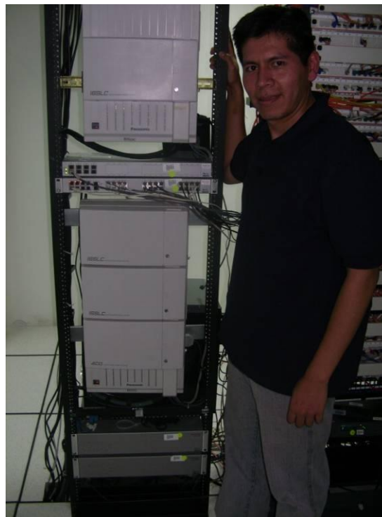
Ing. Arturo Ordoñez, of RUAT, shows the RUAT headquarters communication rack featuring two Xorcom XR3000 servers and two Xorcom Atribanks.
