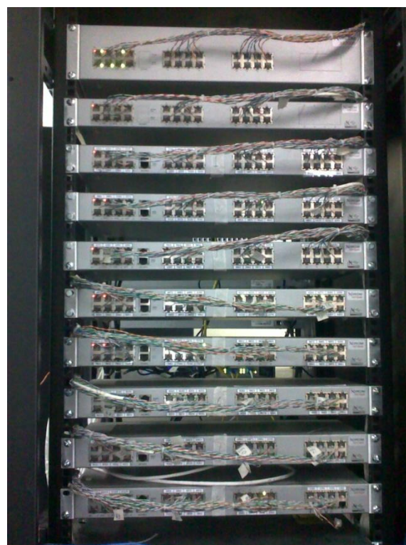
All Xorcom equipment is standard 1U or 2U, 19" rack-mountable for most efficient use of available space.
