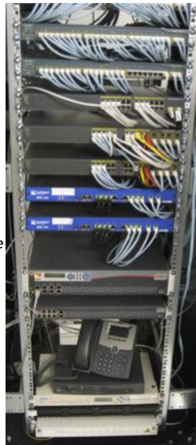
The Modulo solution included a Xorcom IP-PBX with E1 interface and a Xorcom Atribank with analog interfaces.
