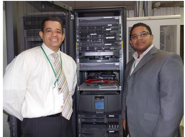
Jose Polanco of AiaTek (l) and Alejandro De La Cruz of Empresas Gasso Gasso S.A. ® next to the communications rack with Xorcom equipment installed.
